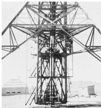
Aerobee rocket standing inside the tower through which it is to be fired.
